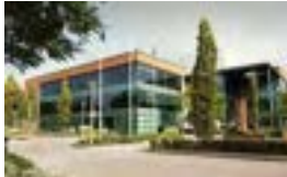
Siemens Belgium TDD Anderlecht Netherlands
