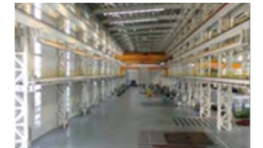
Siemens Morgan Rolling Mill Expansion Shanghai China
