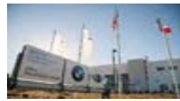
BMW & MINI - NYC Construction Management Services USA
