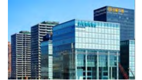
Siemens Centre Shanghai China
