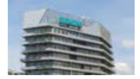
Malaysia CP Tower Consolidation Project - Siemens Energy Malaysia
